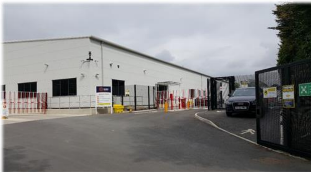
SGN Headquarters on the Longmead Industrial Estate
