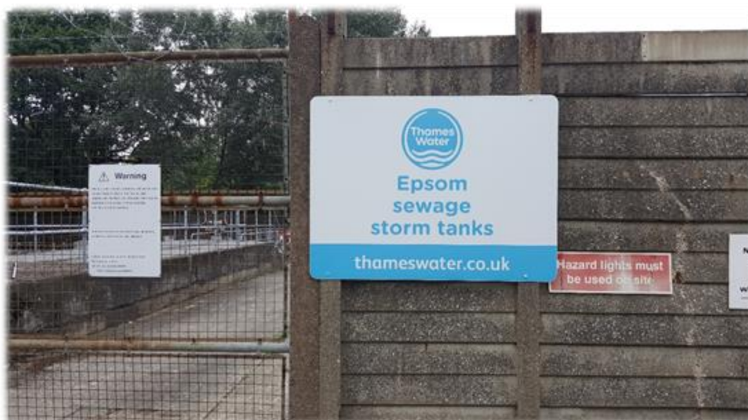
Thames Water sewage storm tanks site
